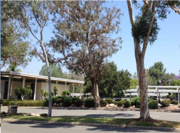
US Bank Solar (Rooftop and Parking Lot)
